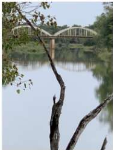
Groblersbrug over the Limpopo River
